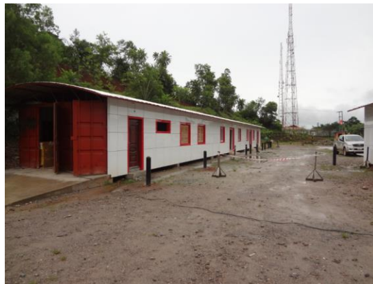
Frequent Power Outages
